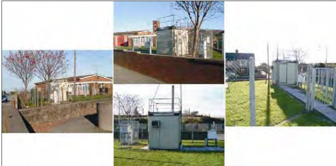
Figure 62: Photos of Fire Station AURN Location ( www.bv-aurnsiteinfo.co.uk )
