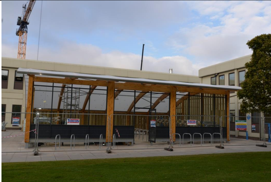
New P/Q block bike shelter under construction, October 2015.
