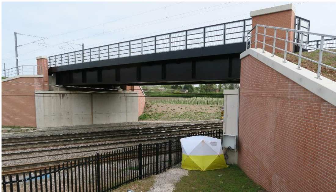
Figure 4. Completed self-sensing railway bridge (west elevation).
