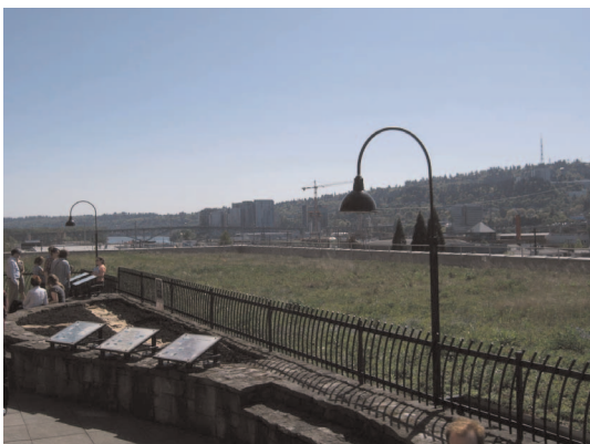
Figure 1. Amy Joslin memorial ecoroof, Multnomah County headquarters building, Portland, Oregon
