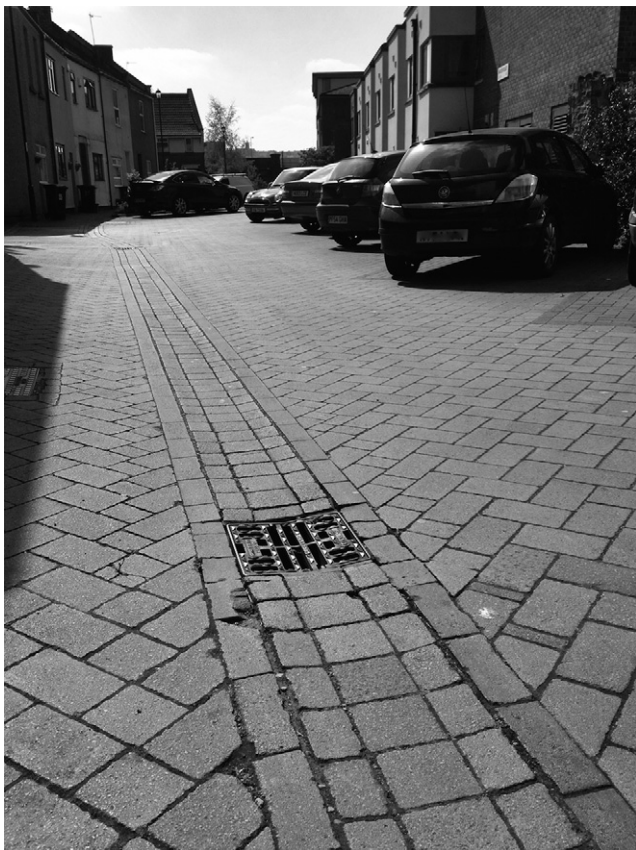
Figure 2. Permeable paving in the UK
