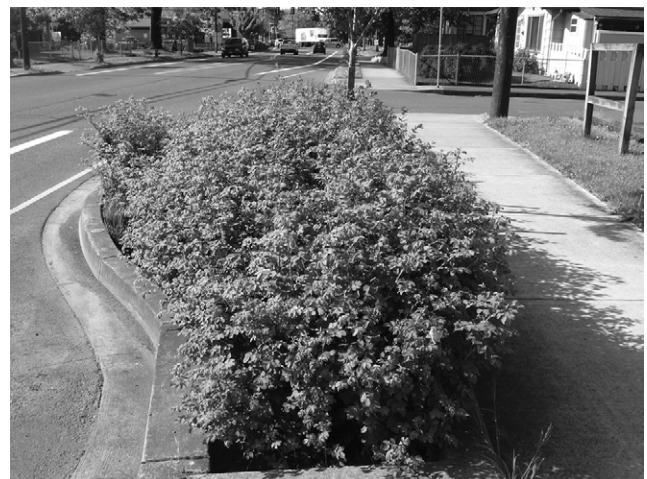
Figure 6. Bioswale with kerb-cut in the USA
