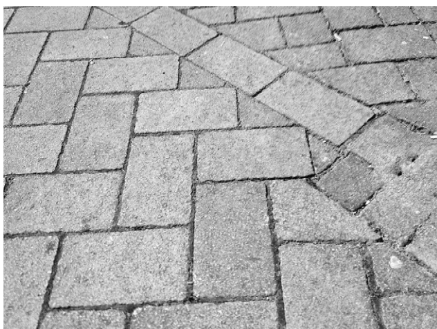
Figure 5. Permeable paving in the UK – close-up
