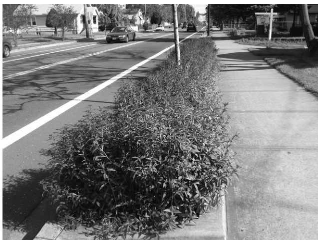
Figure 7. Bioswale without kerb-cut in the USA
