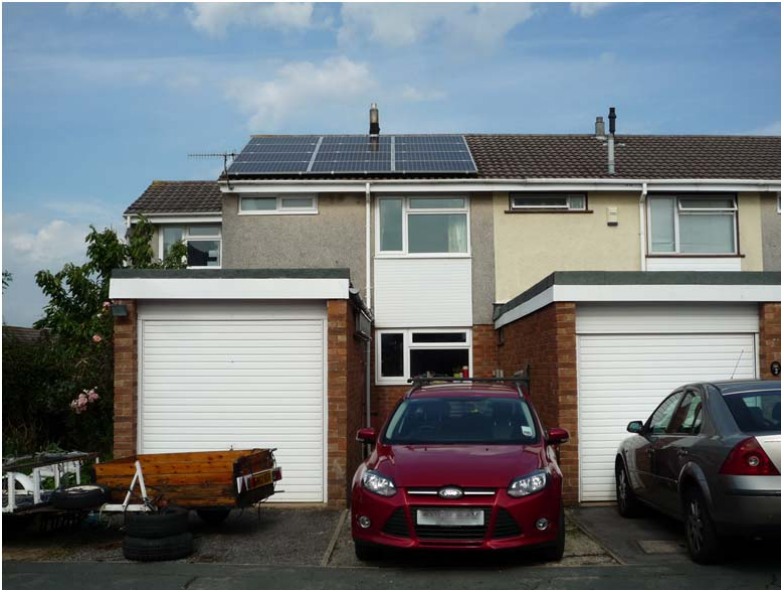
Case019 front elevation including photovoltaic panels
