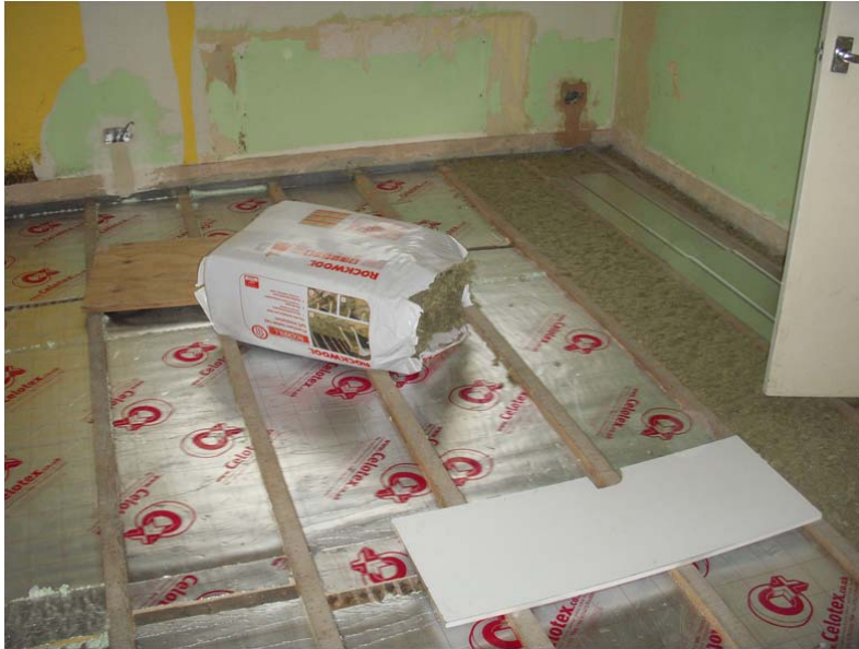
Case006 participant photo of work progression – process of insulating the floors
