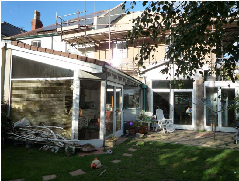
Case016 rear elevation including single storey extension
