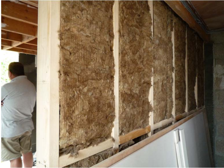
Case007 garage conversion wall insulation
