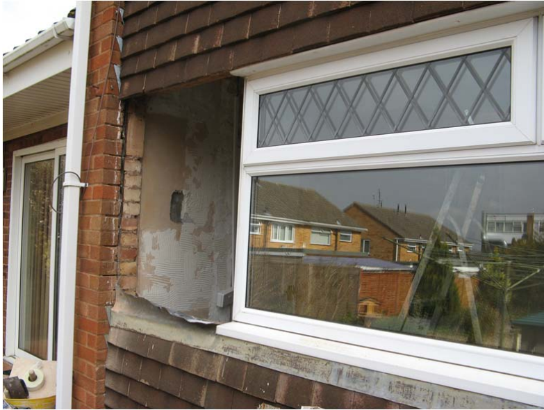
Case013 participant photograph of front window during refurbishment
