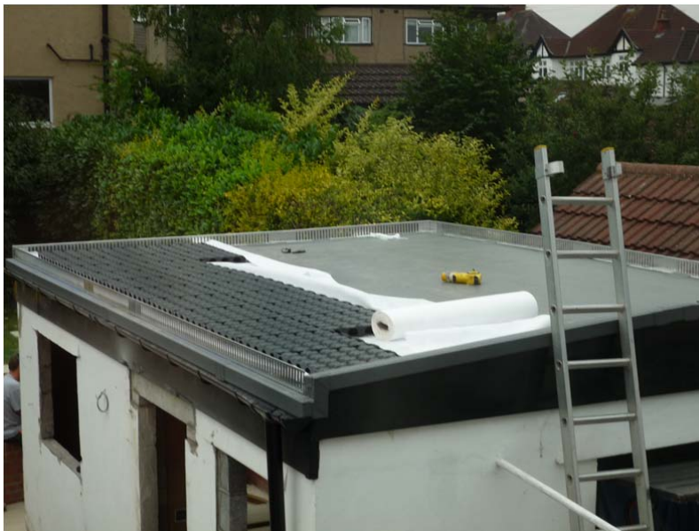
Case007 installation of the green roof
