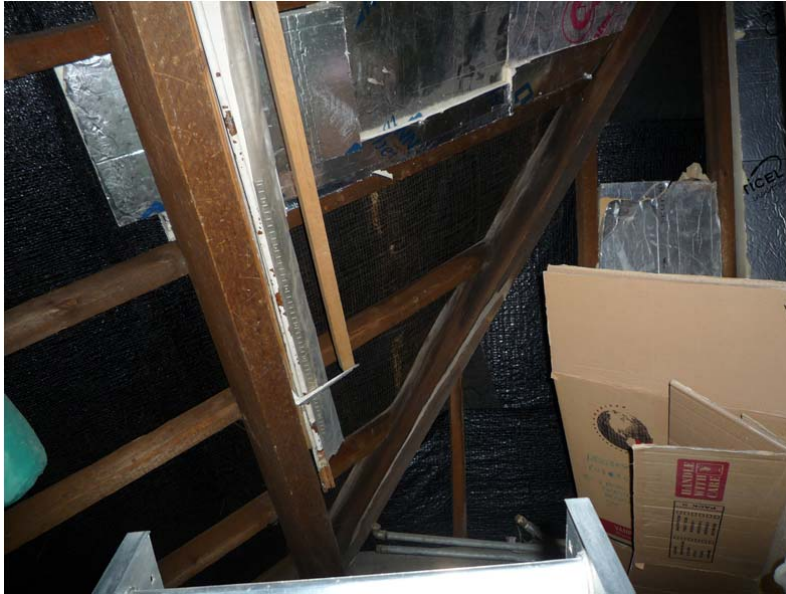
Case021 loft space with partial insulation (rigid) at rafter level
