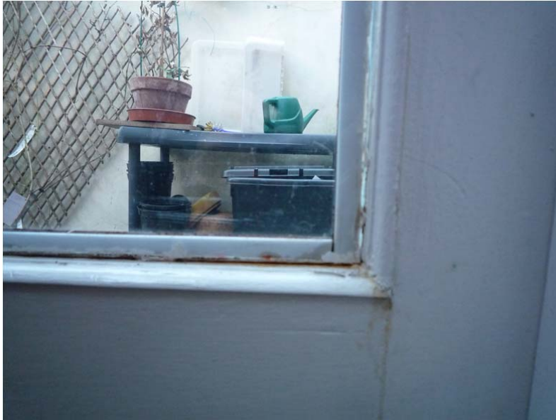
Case018 'do-it-yourself' magnetic, removable secondary glazing
