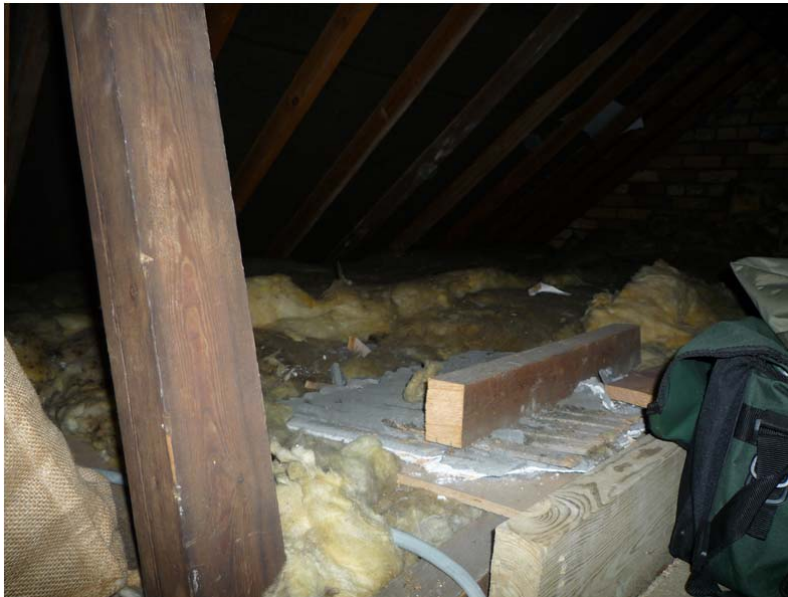
Case011 loft insulation
