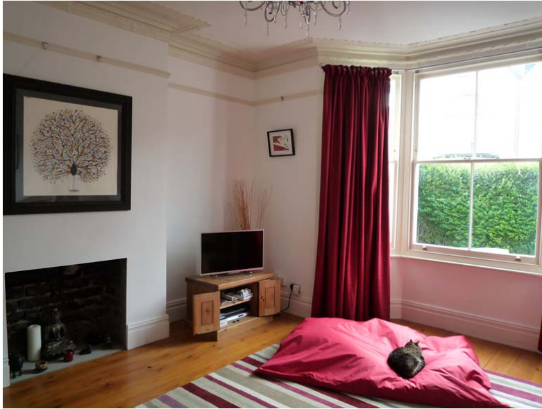
Case008 lounge showing open fire, single glazed sash windows and internal finishes
