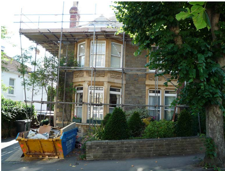
Case016 front elevation including scaffolding for replacement roofing works
