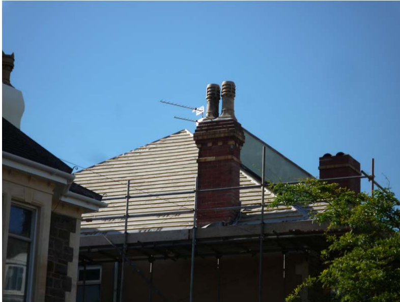
Case016 roofing works
