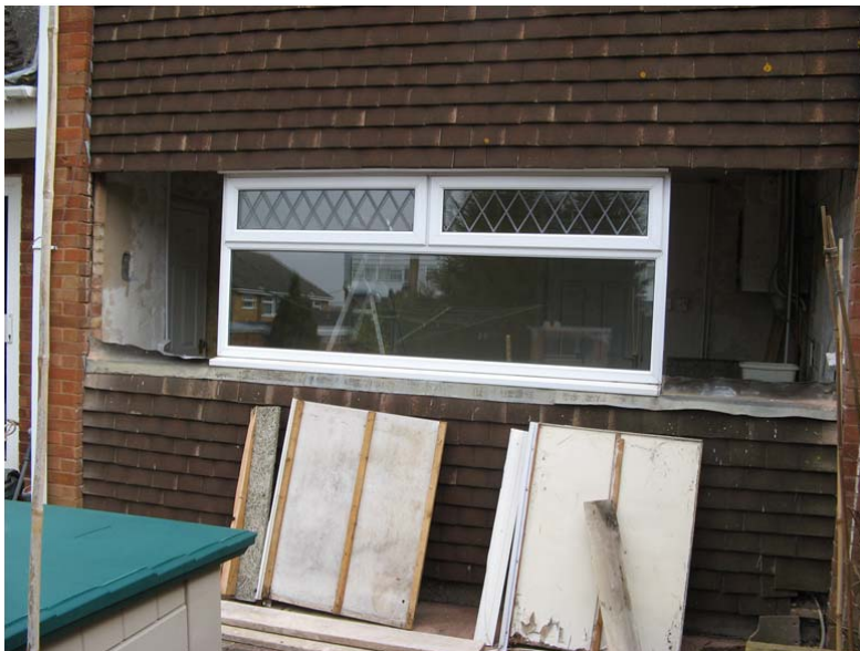
Case013 participant photograph of front elevation during refurbishment
