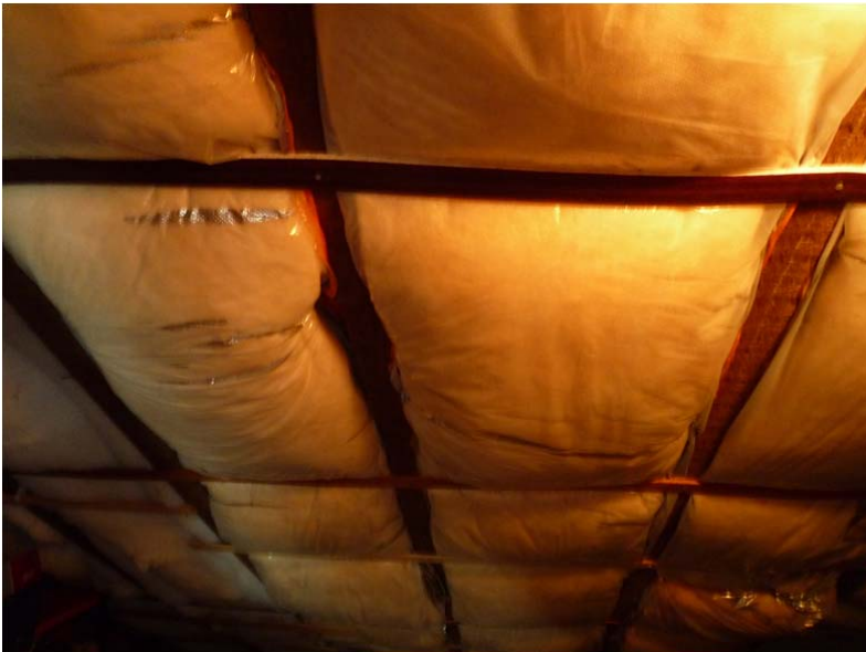
Case009 loft insulation at rafter-level
