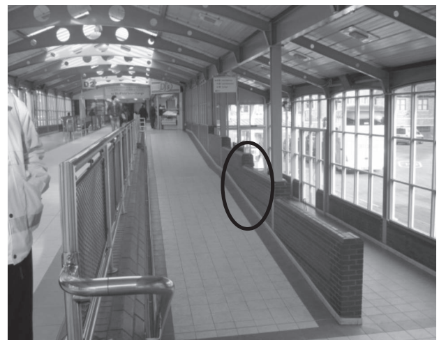
Figure 7. Handrails were only provided on one side
