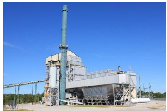
Aspen Power plant in Lufkin, TX
