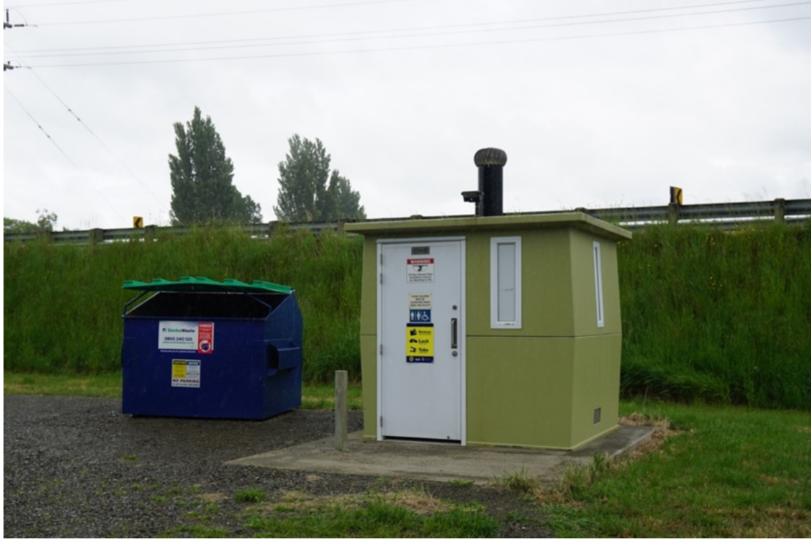
Figure 4.4: Chamberlains Ford freedom camping facilities-vaulted toilet and large waste disposal. Source: Author
