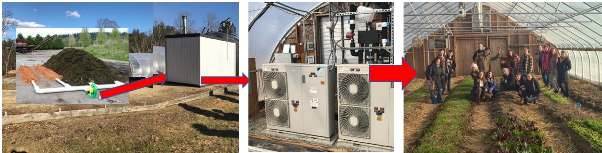
Figure E.2 A simplified ASP/HRC system like the one pictured (Left) would be placed on the sandy pad area behind this high tunnel. Vapor would be piped through the structure housing the insulated water tank to increase water temperature in the tank. The existing heat pumps in the structure would draw on this warm water source to operate at high efficiency in producing warm air for the structure.
