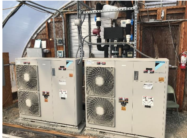
Figure E.1 Left: Image of a high tunnel at Woodman Farm with insulated water heat storage tank used to capture heat removed from the structure and then as a source for the heat pumps within the structure. Right: Two reversible air-to-water heat pumps inside the high tunnel pictured at left. See text for additional explanation.
