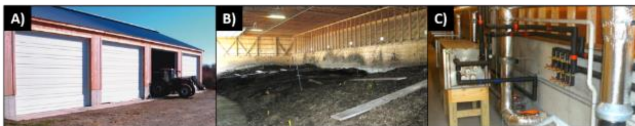
Figure 3.2 Joshua Nelson Energy Recovery Compost Facility located at the University of New Hampshire Burley-Demeritt Organic Dairy Research Farm in Lee, New Hampshire, USA. The images show A) the exterior doors to the facility where compost feedstock is loaded, B) piles of composting material in the facility, and C) the back of the facility where the gas exhaust from the facility is piped, allowing for heat recovery and measurements.
