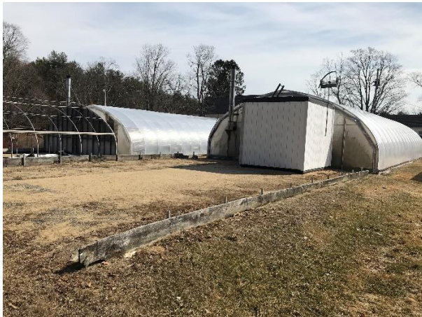
Figure E.1 Left: Image of a high tunnel at Woodman Farm with insulated water heat storage tank used to capture heat removed from the structure and then as a source for the heat pumps within the structure. Right: Two reversible air-to-water heat pumps inside the high tunnel pictured at left. See text for additional explanation.
