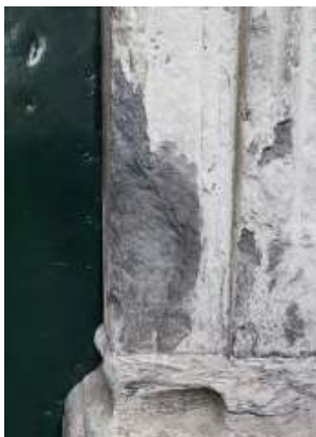
Fig.9 - Loss of components due to mechanical damage
