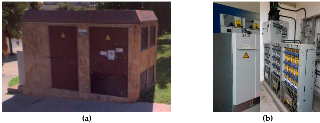
Figure 1. Distribution Center example. (a) Outside view, (b) Inside view.
