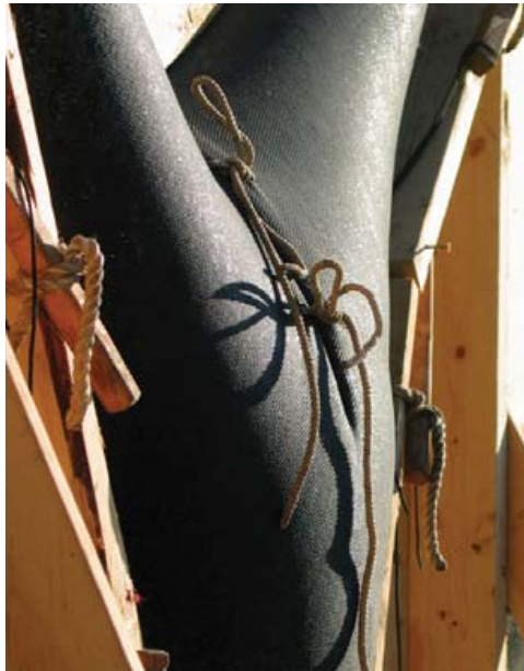
Figure 2: Photo of a textile formwork 1 .
