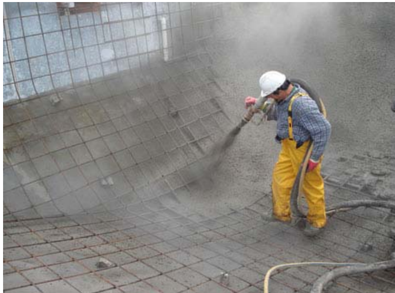
Figure 3: Photo showing spray applied concrete.
