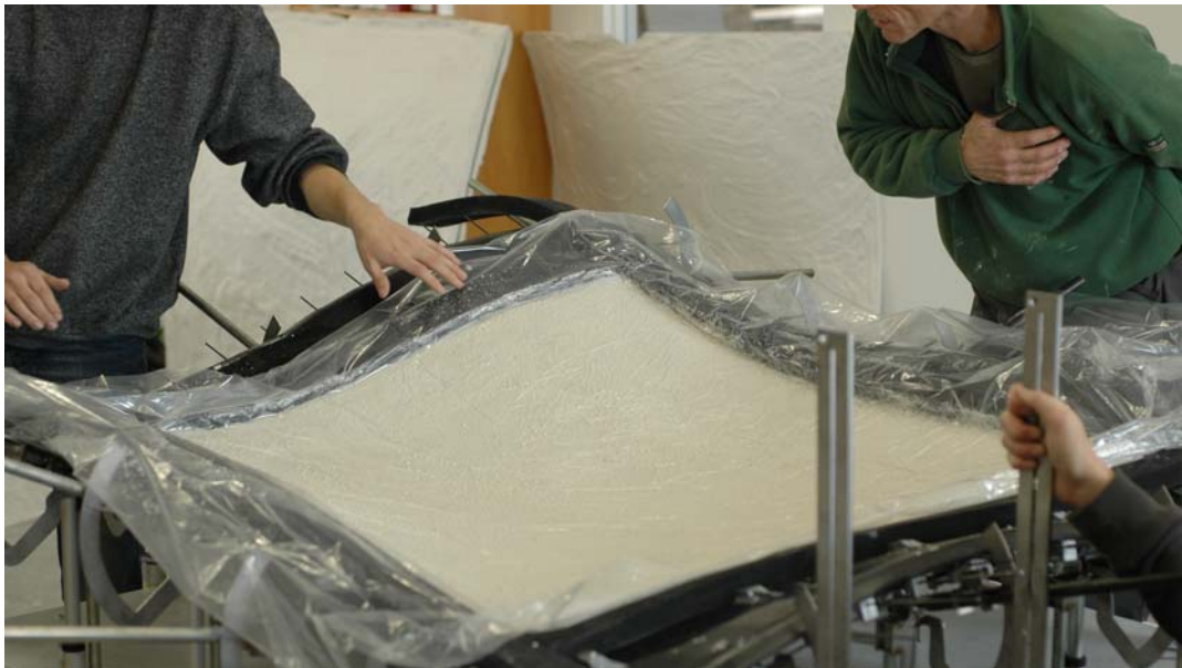
Figure 9: Casting of a double curved fiber reinforced concrete panel.
