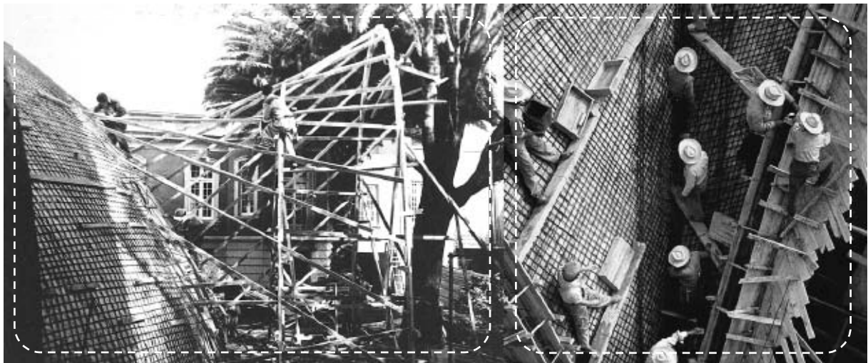
Figure 4: formwork construction by Felix Candela 2
