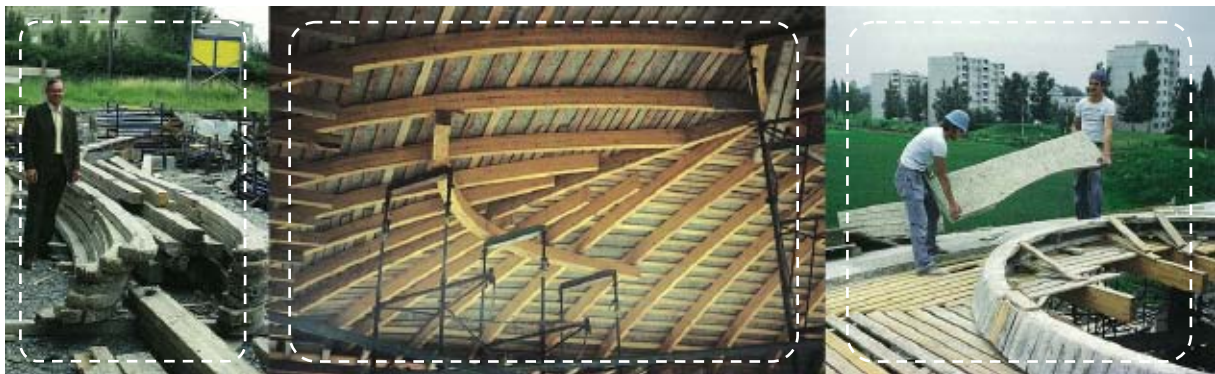
Figure 6: formwork system by Heinz Isler 6
