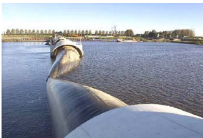
Figure 9: V-notch in gas filled dam
