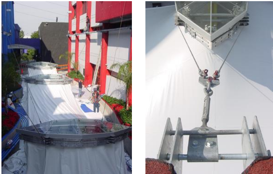
Figure 6: Installation and detail of fittings for assembly
