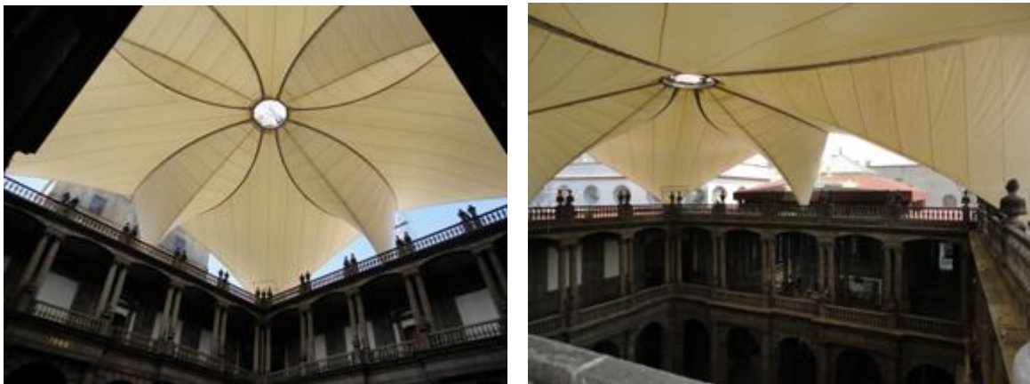
Figure 1: Interior view of the tent structure over the central courtyard of the Palacio de Minería building.
