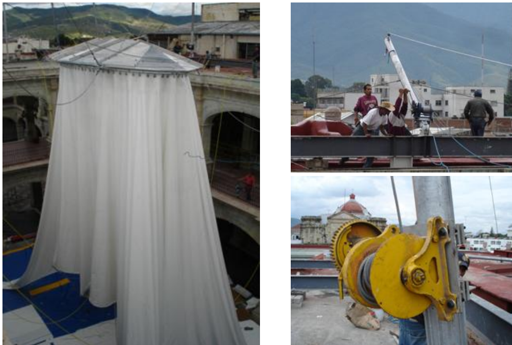
Figure 9: Installation and detail of the lifting system.
