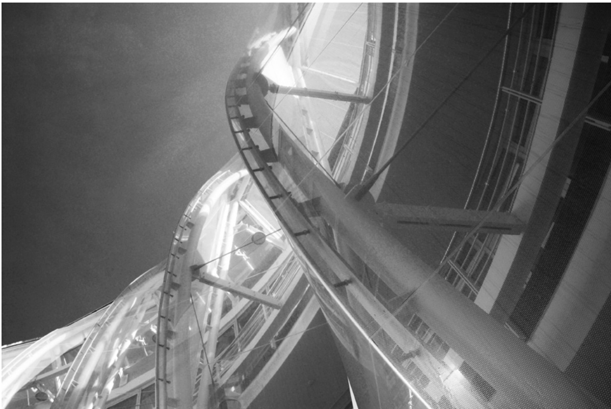
Figure 2: Second skin façade of the Centre for Gerontology, Bad Tölz (Source: Jan Cremers)
