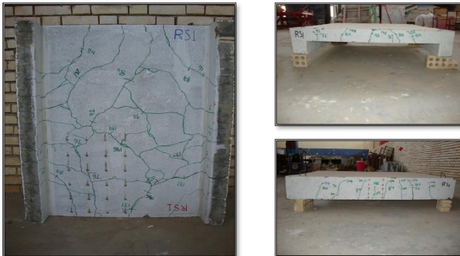
Fig.(3): Cracking Pattern at Failure for Model (S6)
