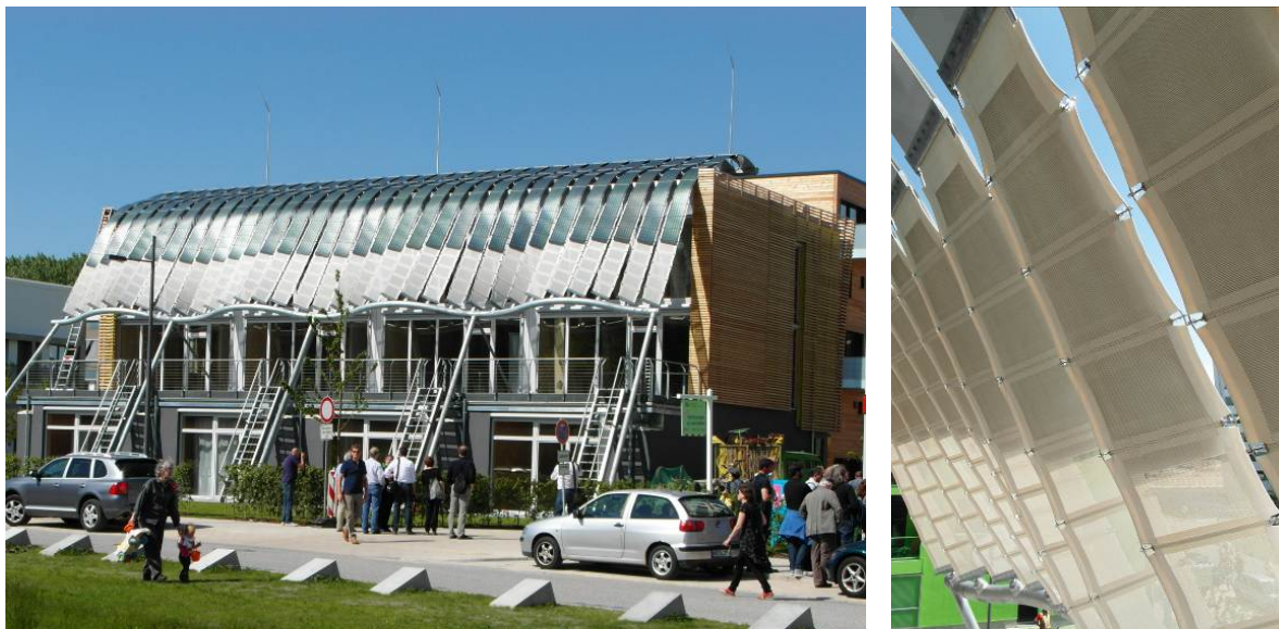
Figure 8: Finished 'Softhouse' building with multifunctional adaptive facade at IBA Hamburg Mai 2013
