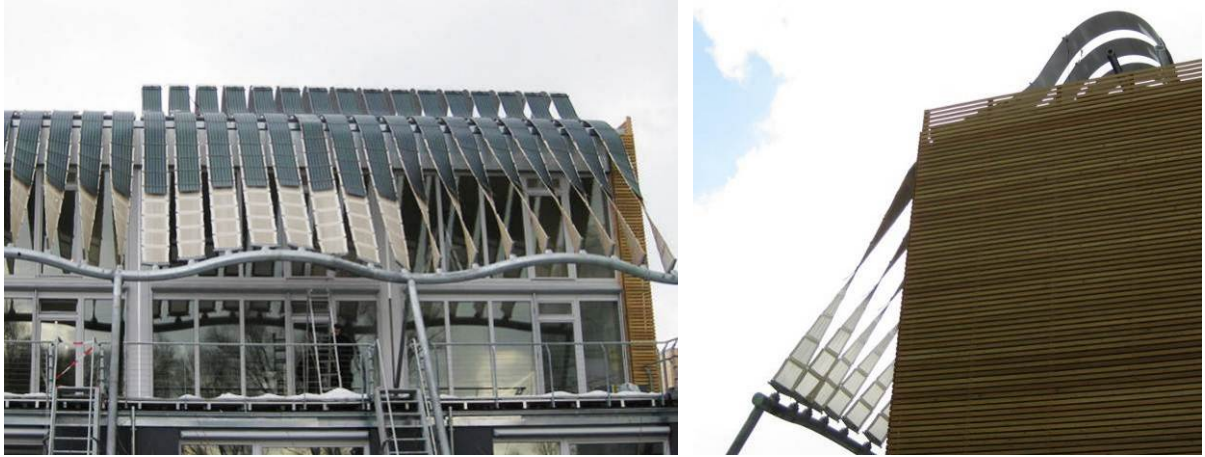
Figure 7: Testing various modes of shape adaptation on the finished structure (Pictures by Textilbau GmbH)
