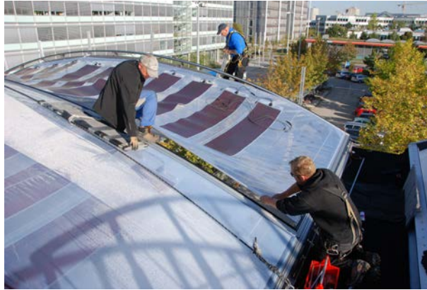
Fig. 6 - Fixing the last cushion in place
