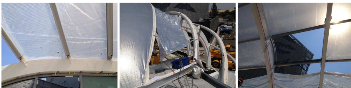
Figure 13: Installation phase of the pneumatic envelope (Source: Canobbio)
