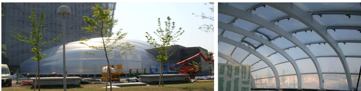
Figure 12: Pictures of the realization, from outside and inside (Source: Canobbio)
