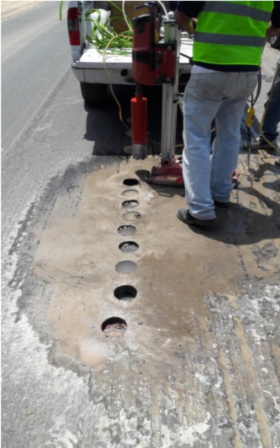
Figure 16. Extraction of cores.
