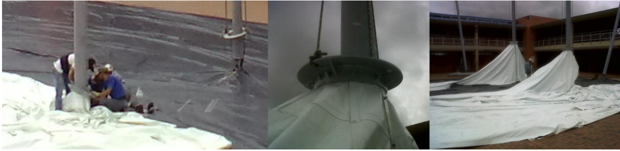
Figure 9: Membrane elevation process
