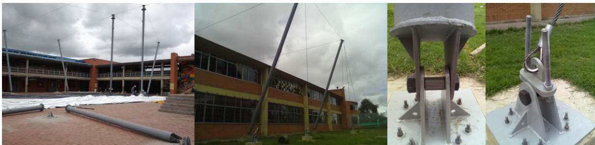
Figure 8: Assembly process structure, masts, anchor plates and cables
