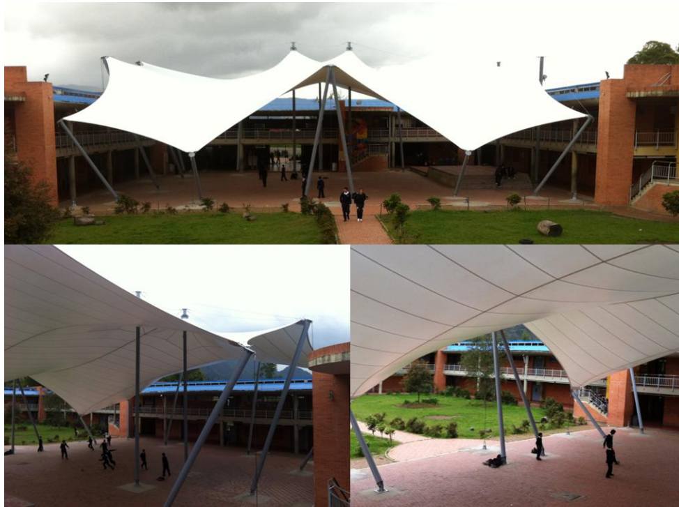
Figure 7: Front and inside of the structure
