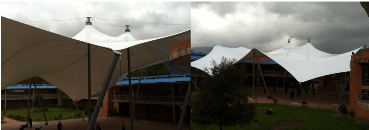
Figure 20: Positioning the membrane anchor points, tensioning end
