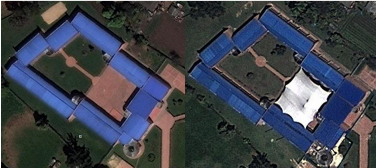
Figure 1: Air photography. Central courtyard uncovered and covered
