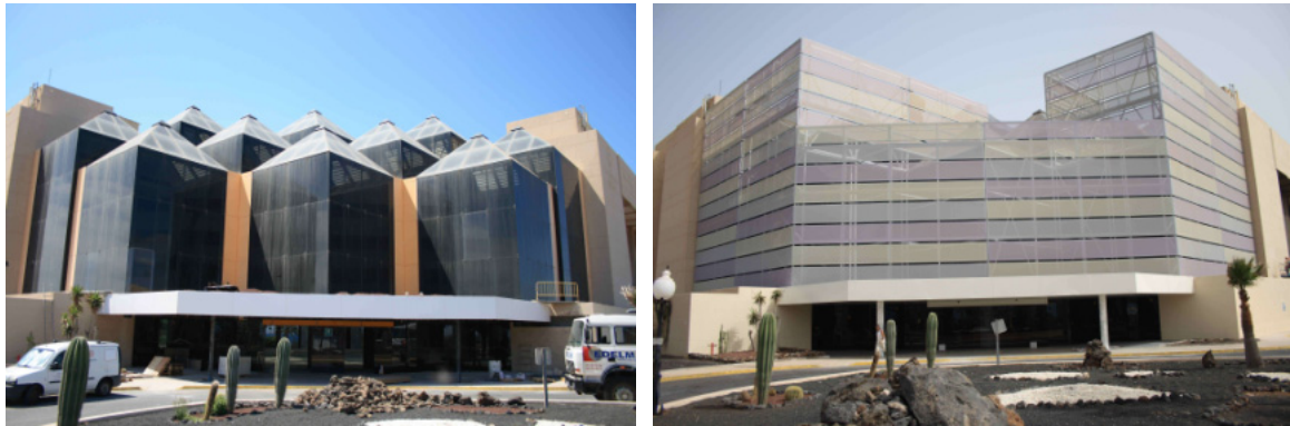
Figure 1: Hotel Oasis façade, before and after the textile façade installation.
