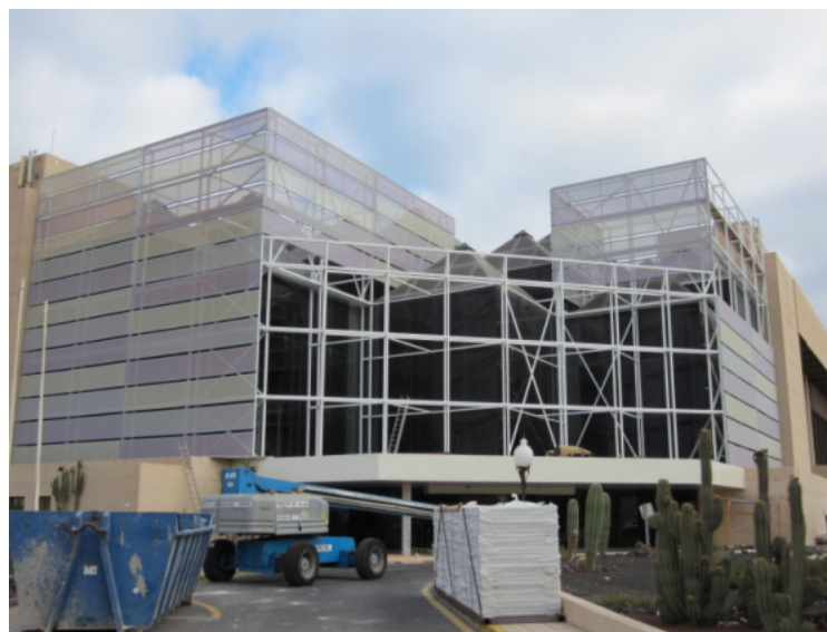
Figure 9: Secondary steel structure and textile façade under installation
