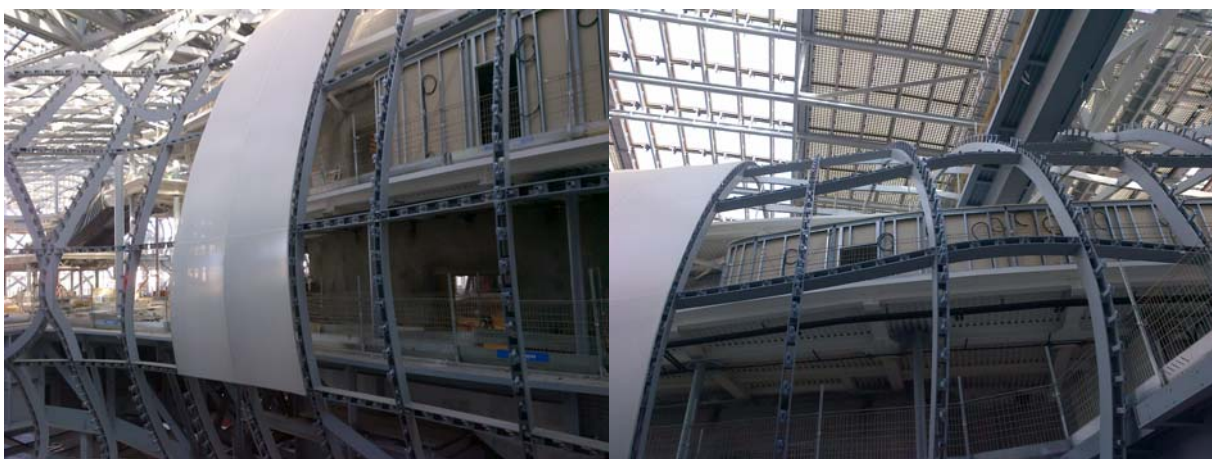
Figure 18: steel grid and first panels
