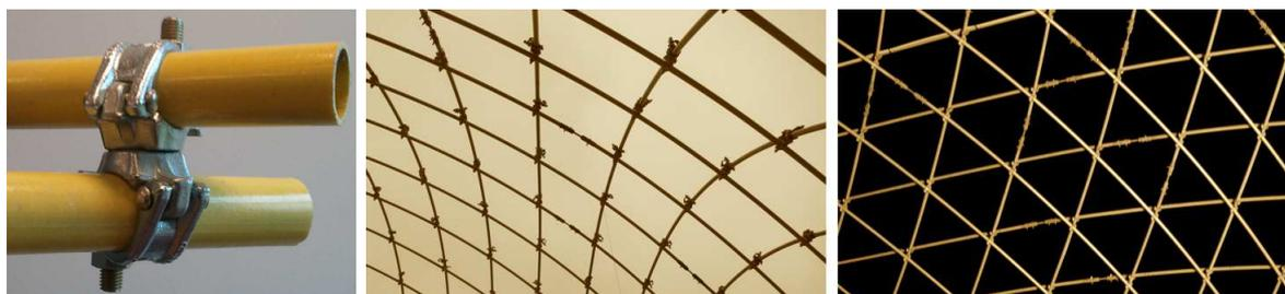
Figure 7: a. Joint detail. b. Mesh before bracing. c. Mesh after bracing.
