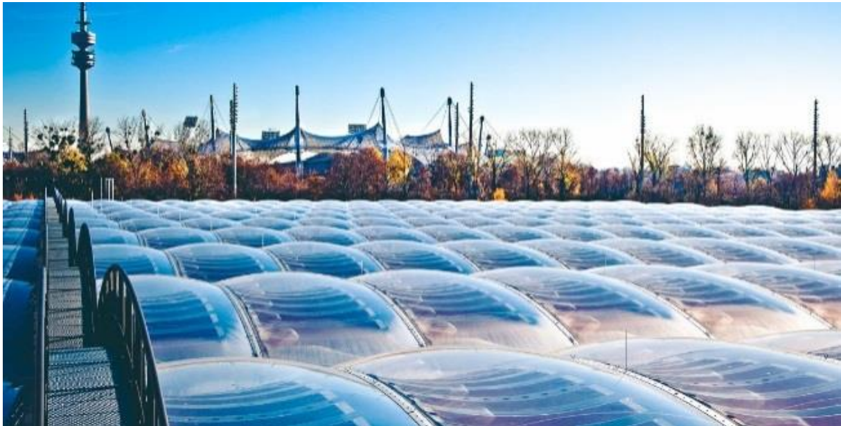
Figure 2: Municipal Waste Management Department parking cover, Munich (Germany), triple layer ETFE cushions incorporated with photovoltaic cells, completed in 2011.
