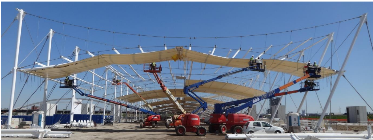
Figure 11: View of the Decumano during installation
