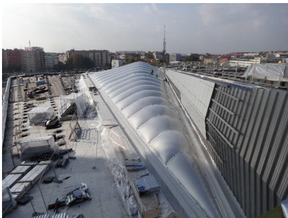
Figure 4: Top view of the ETFE skylight.
