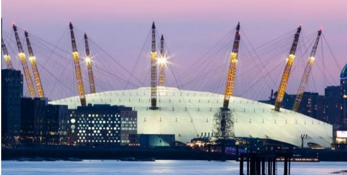
Figure 1: Millennium Dome Greenwich, London (UK), PTFE coated fiberglass fabric, completed in 1998.
