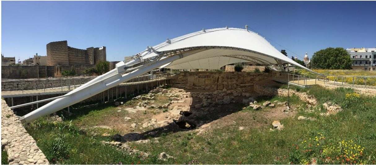
Figure 6: View of the PTFE roof from outside (Tarxien temple site)
