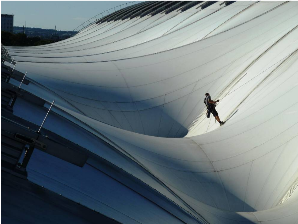
Figure 24 Main station Dresden, partial view of roof with funnels
