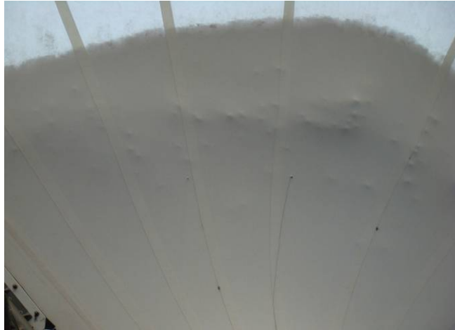
Figure 27 Main station Dresden, clumped snow in funnel with local peaks
