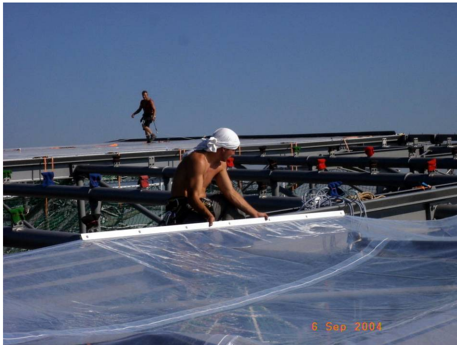
Figure 11 Keder profile is pushed onto the edge of an ETFE foil
