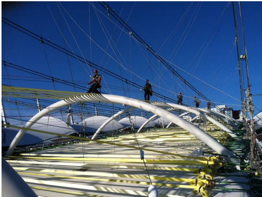
Figure 13 Membrane arches prepared for lift of membrane
