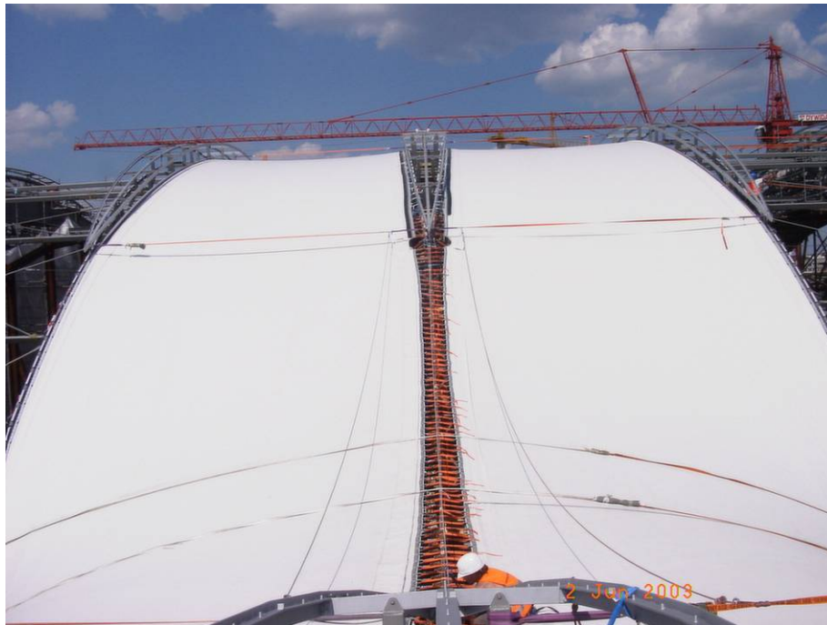
Figure 5 Battery of ratchet belts for tensioning of two adjacent membrane bays
