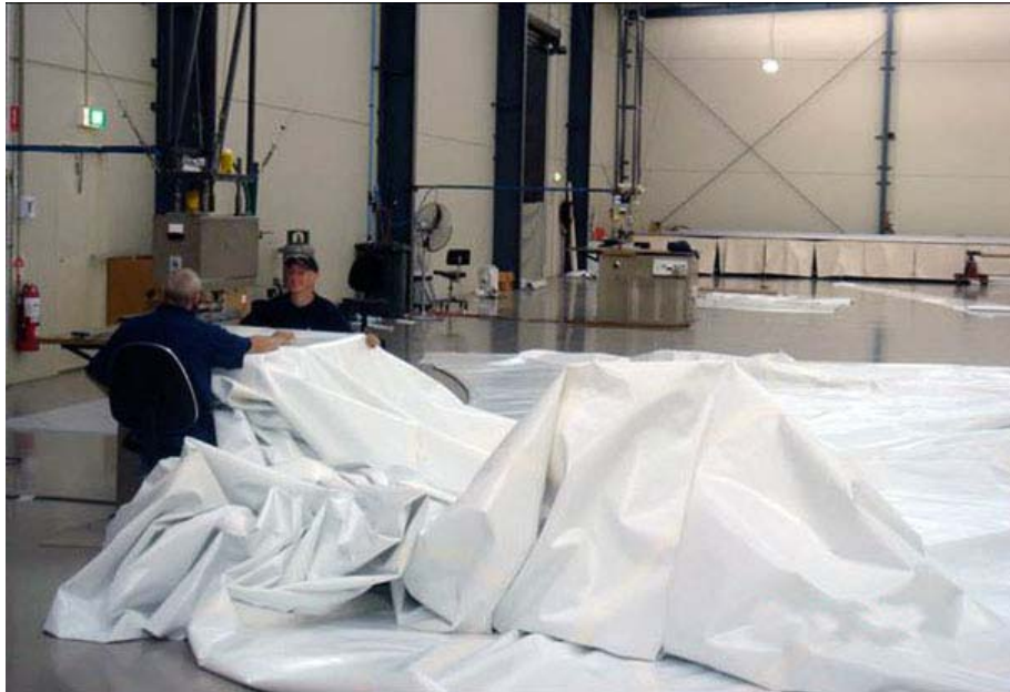
Figure 2 Welding of Polyester-PVC fabric with high frequency welding machine (Photo: CenoTec)
