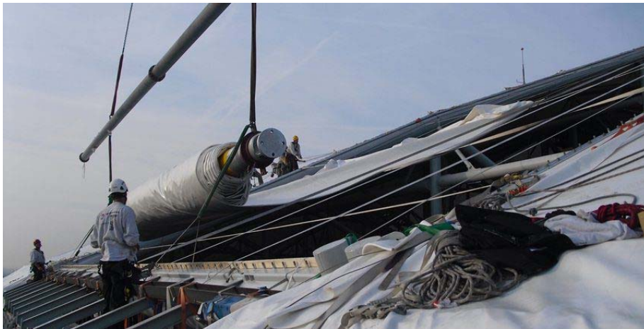
Figure 14 Unrolling of membrane with use of crane traverse (Photo: Montageservice LB)
