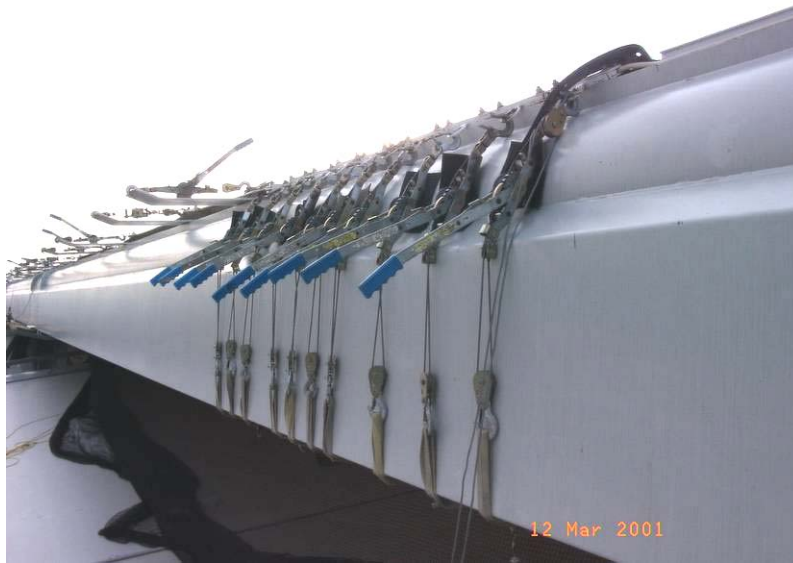
Figure 18 Battery of tirfers to tension a membrane bay
