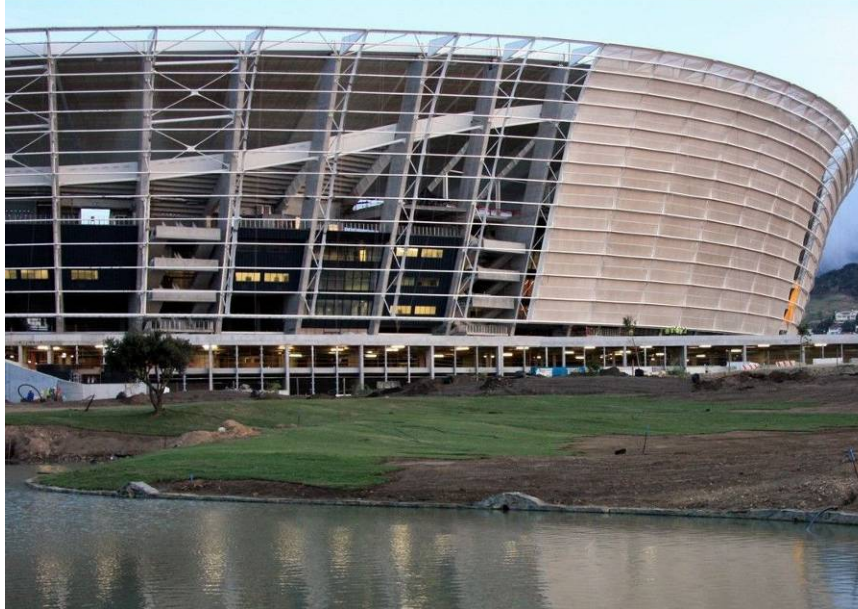
Figure 28 Green Point Stadium, facade during installation
