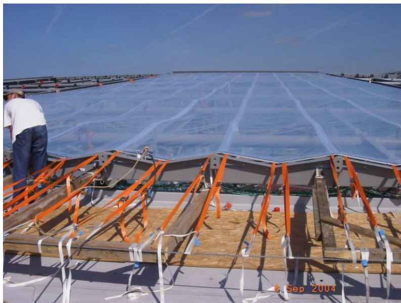
Figure 19 Tensioning of a single layer ETFE-foil
