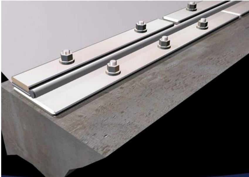
Figure 9 Clamping edge, bolted to concrete structure (© Birdair)
