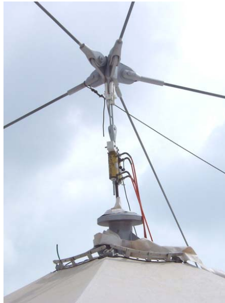
Figure 6 High point of a membrane panel during tensioning with hydraulics (© form-TL)
