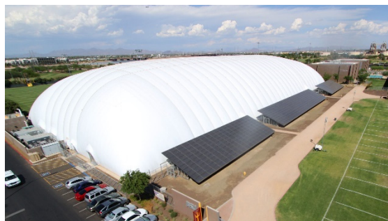
Figure 2. Air-supported structures («The Verde Dickey Dome»)
