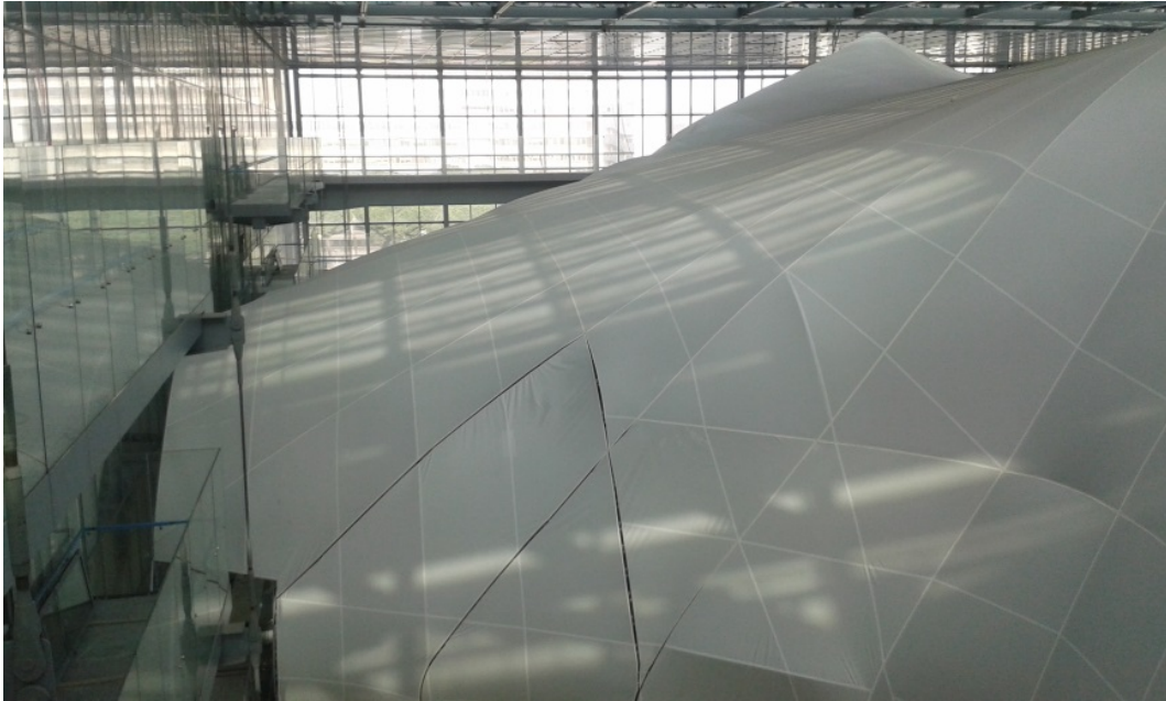
Figure 18: open joints during installation
