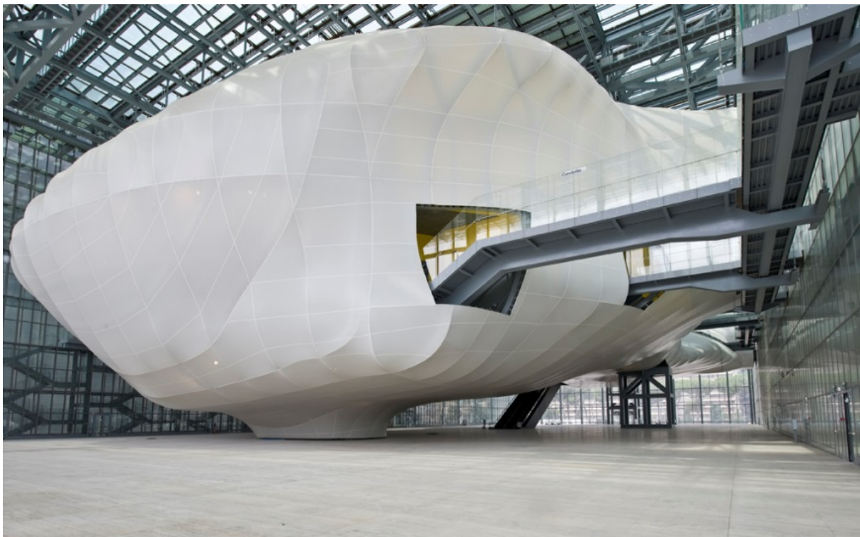
Figure 19: outside view zone 5
