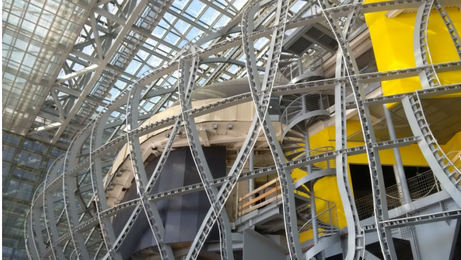
Figure 16: steel structure with installed secondary structure
