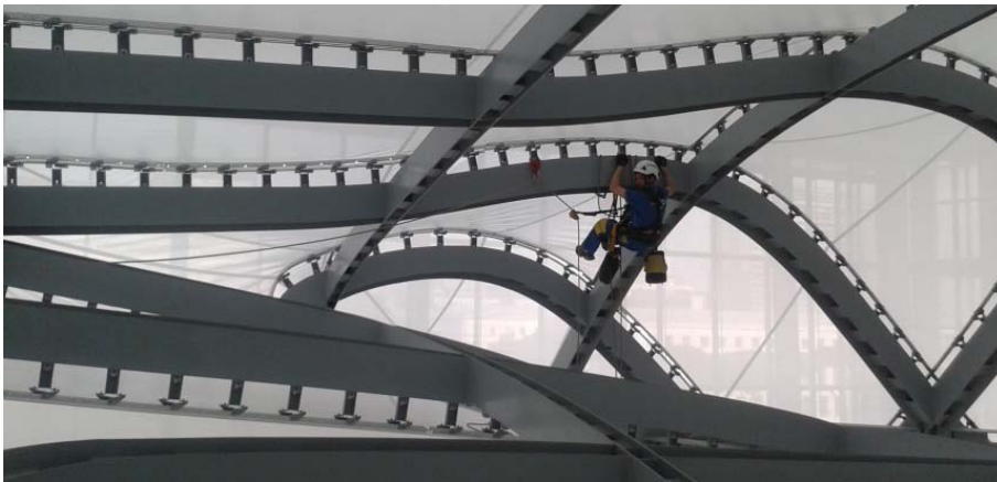
Figure 17: installation from inside
