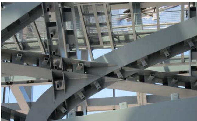
Figure 6 / Figure 7: stud detail of the steel structure / isometric view attachment and push up detail
