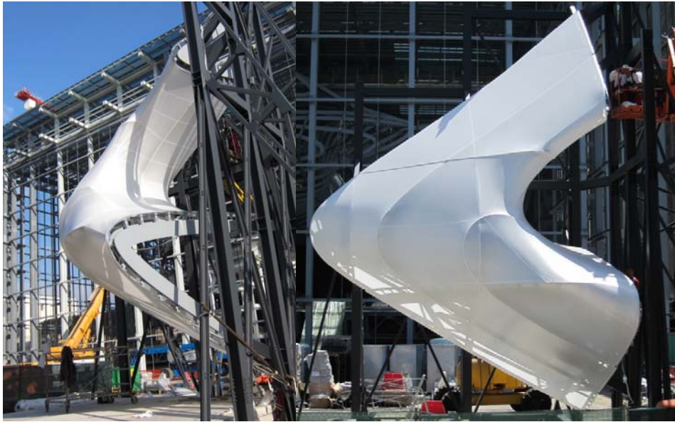
Figure 4 / Figure 5: First tensioned membrane mock-up / Second tensioned membrane mock-up
