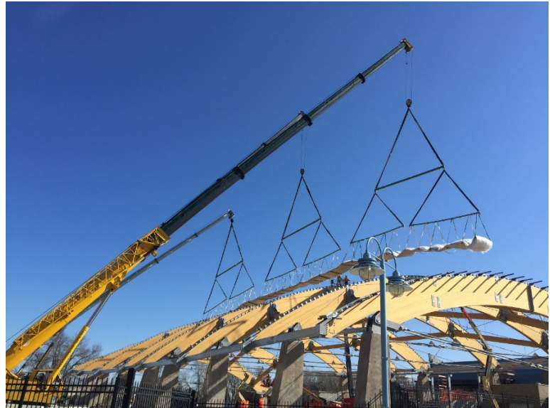
Figure 12: Three cranes with spreader bars placing fabric
