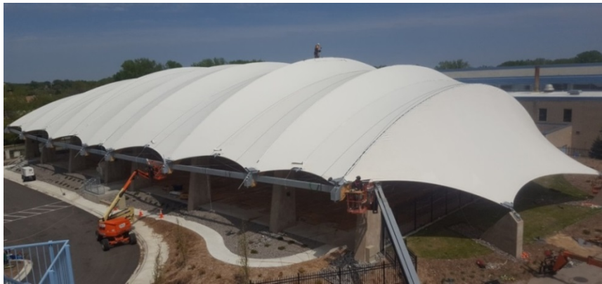
Figure 2: The roof structure nearing completion
