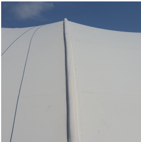
Figure 13: Fabric closure at arch top
