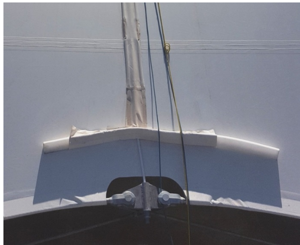
Figure 14: Valley closure / diverter intersection
