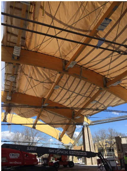
Figure 11: Fabric reinforcements during erection
