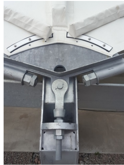
Figure 10: Typical "floating" membrane plate
