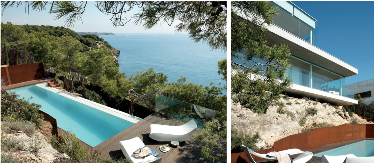
Figure 4. Southeast façade and swimming pool, views to the sea horizon, ©Jordi Miralles / Figura 4. Fachada sudeste y piscina, vistas hacia el horizonte marino, ©Jordi Miralles.
