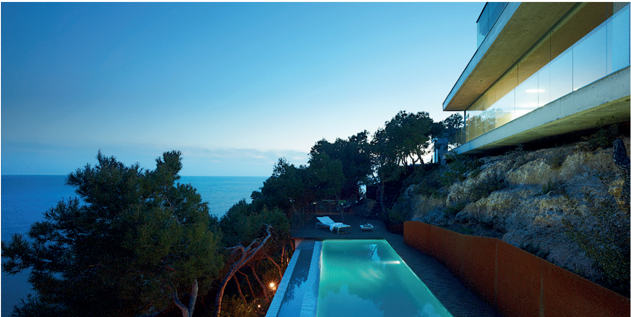
Figure 1. The house on the cliff, southwest view, 2006, ©Eugení Pons / Figura 1. Casa en el acantilado, vista a sudoeste, 2006, ©Eugení Pons.
