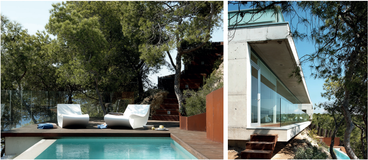
Figure 3. Southeast facade and swimming pool, integration with the landscape, ©Jordi Miralles / Figura 3. Fachada sudeste y piscina, integración con el entorno paisajístico, ©Jordi Miralles.
