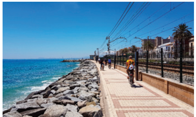
Figure 3. Bike path and railway in Premià de Mar
