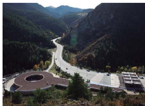
Illustration C, aerial view of the Cadí tunnel
