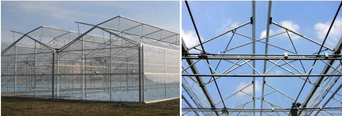
Figure 15. ETFE covered greenhouse (AGC Chemicals, 2019).
