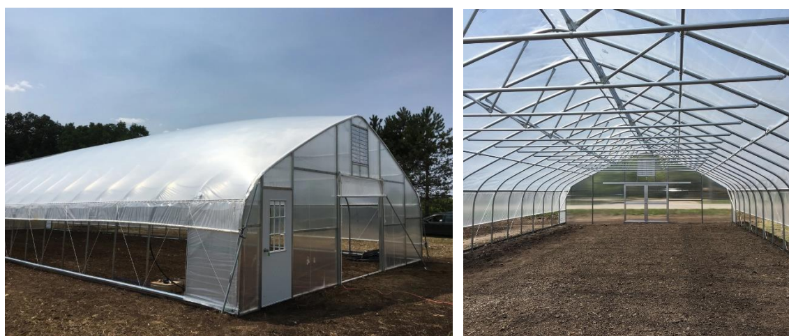
Figure 13. Double layer polyethylene cover greenhouse (Tunnel Vision Hoops, 2019)
