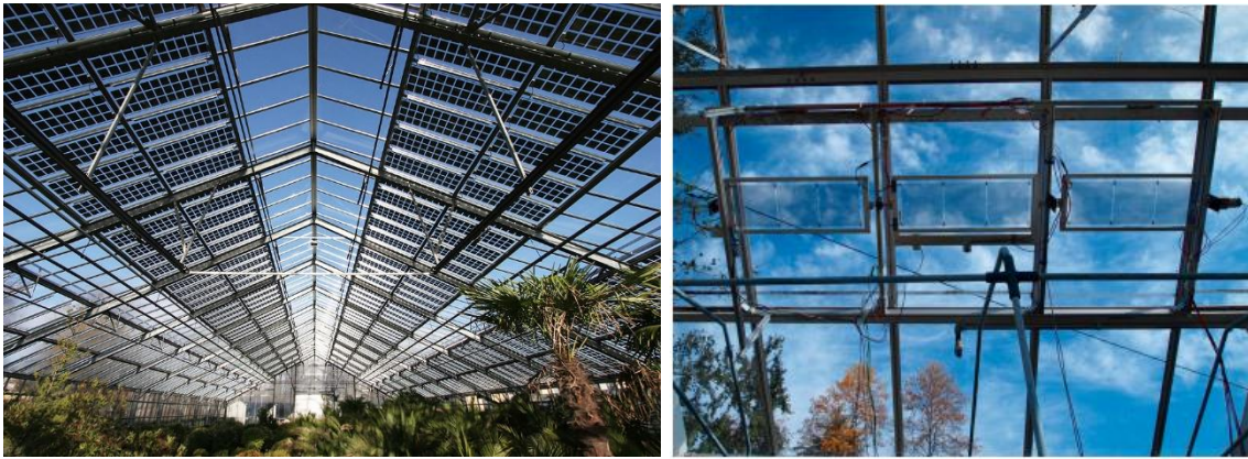
Figure 16. On the left, inside of a greenhouse with a solar cover of conventional panels. On the right, a semi-transparent panels with Sphelar® Technology (Cossu et al., 2016)
