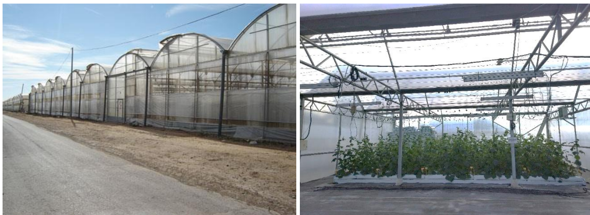
Figure 12. Polyethylene covered multitunnel greenhouse in Almeria (left) and IRTA Cabrils - Polyethylene covered greenhouse (right) (Montero et al., 2011; Ribas, 2019)
