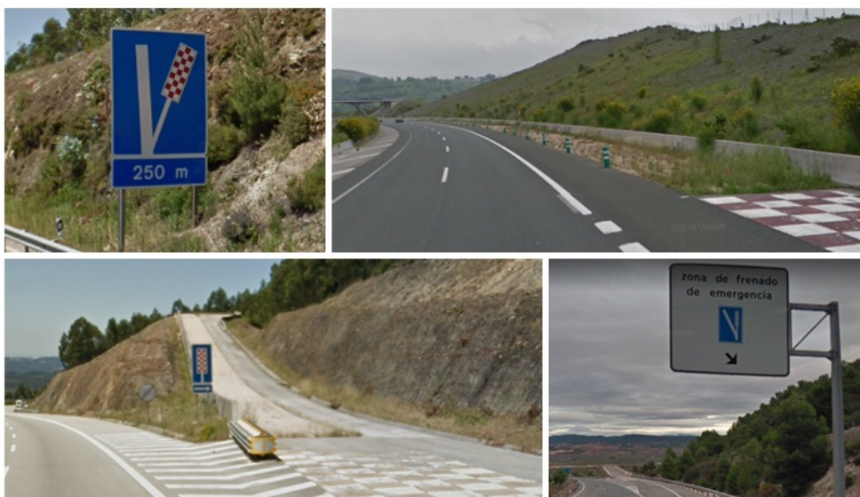
Figure 16: Some examples of runaway ramps and the road sign that informs about the existence of a runaway ramp. Note that such sign may also show some format variations between countries. GOOGLE MAPS.
