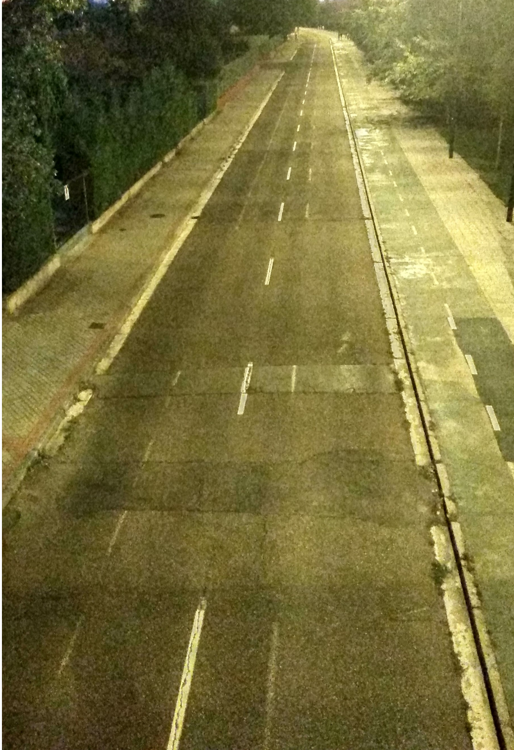
Figure 4: Example of a street in Valladolid (Spain) whose former road markings have not been completely erased. Notice that the two lanes have been broadened by terms of eliminating the former on-street parking space, which was placed at the leftmost side of the road. The set of road markings formed by the former (on-street parking and former road edge) and the newer lines (real road edge) could become a barrier for Lane Support Systems.
