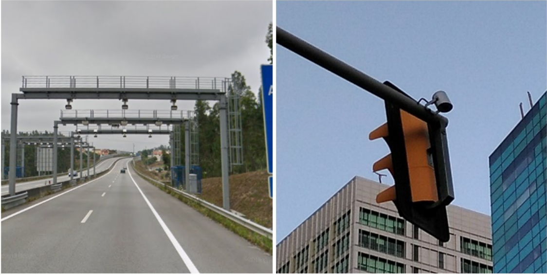
Figure 25: Some road sensors such as license plate recognition cameras (placed in gantries for tolling systems and average speed controlling) or other traffic cameras (for traffic management) are currently being used at major streets and road sections.
