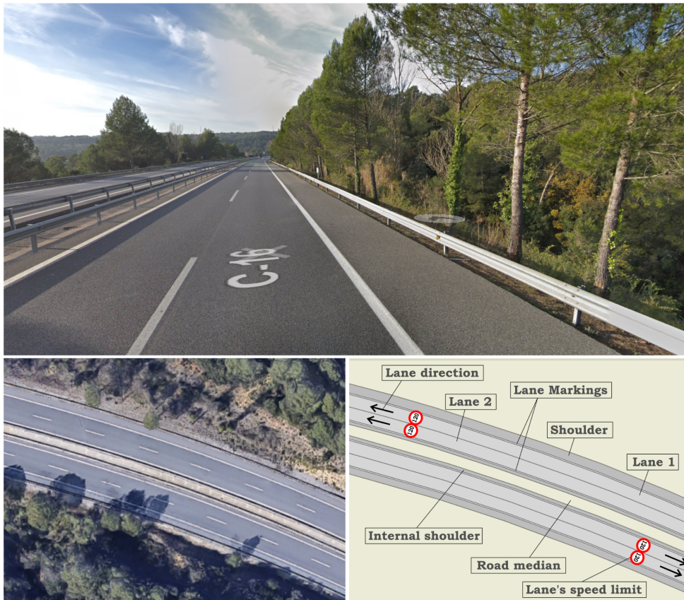
Figure 15: The precise marking, positioning and definition on digital maps* of the existing refuge bays and shoulders would be a quite important requirement in order to ease vehicles to safely, carefully stop in any case it were required. GOOGLE MAPS / OWN ELABORATION.
