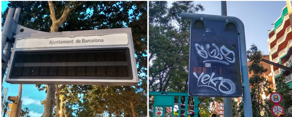
Figure 17: Variable message signage panels in Barcelona. Notice that the panel represented at the figure on the left side is not displaying any information and the right panel seems to be malfunctioning beyond being vandalised. OWN ELABORATION.
