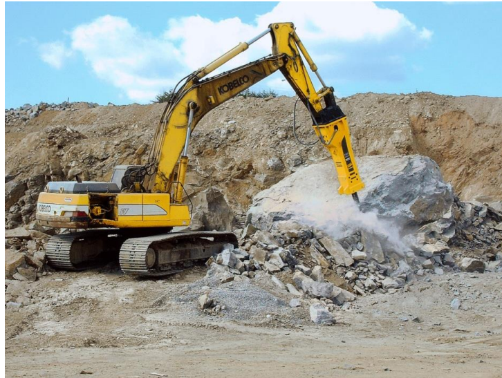
Figure. 3.4 Boom mounted breaker ( http://mcquaidengineering.com 2019).
