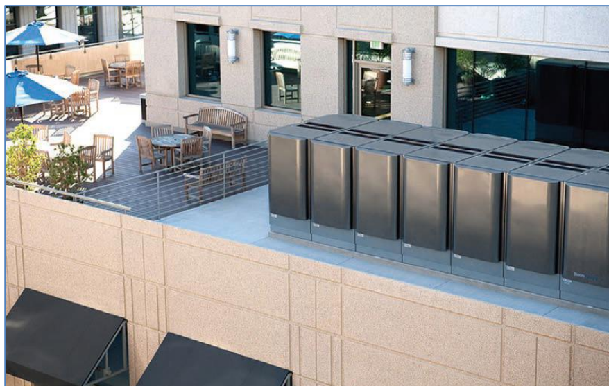
Figure 13. Modular SOFC system for CHP in a building from USA firm Bloom Energy. Several modules are combined to meet the required power. [15]
