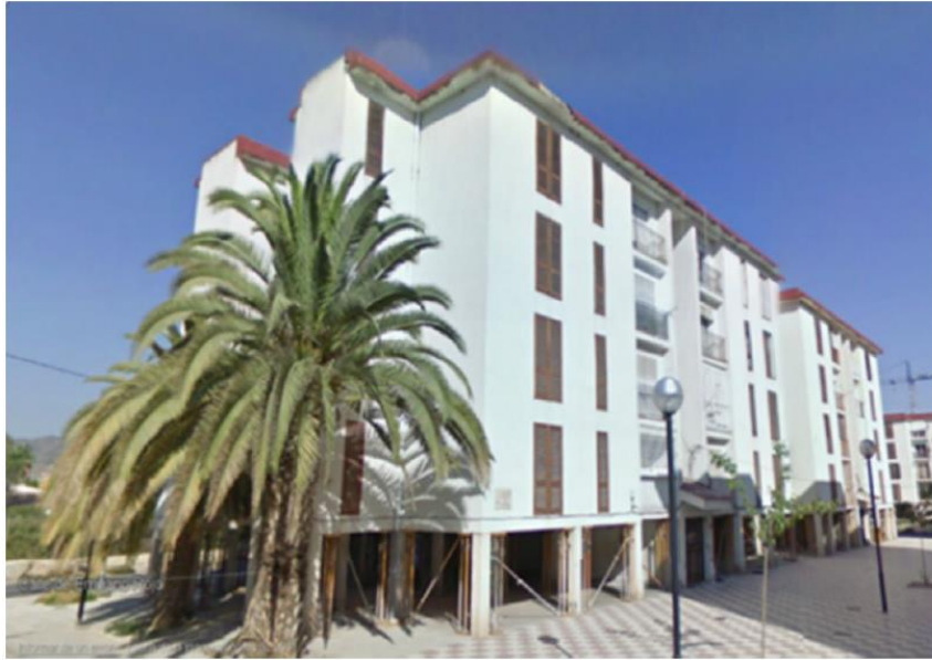
Figure 3. Buildings located in the San Fernando neighbourhood of the city of Lorca, Spain, affected by the earthquake.
