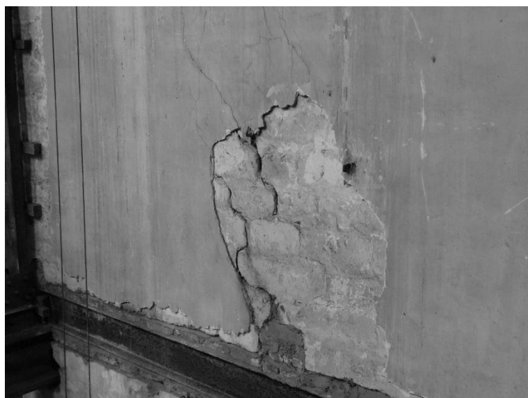
185 Figure 3 Close-up of cracks 4 on main nave wall (photo by Els Verstrynge, 2018).
