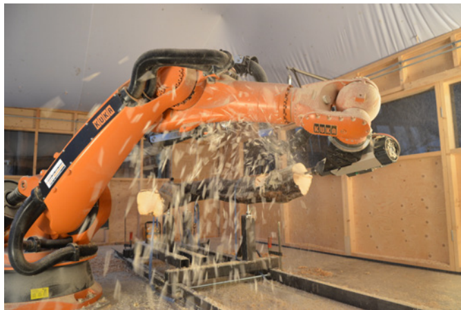
Figure 14: Subtractive fabrication of connections in irregular forked timbers using a router mounted on a 6-axis industrial manufacturing arm (Mollica and Self, 2016, Devadass et al., 2016). Photograph by Swetha Vegesana. Courtesy of the Architectural Association School of Architecture.
