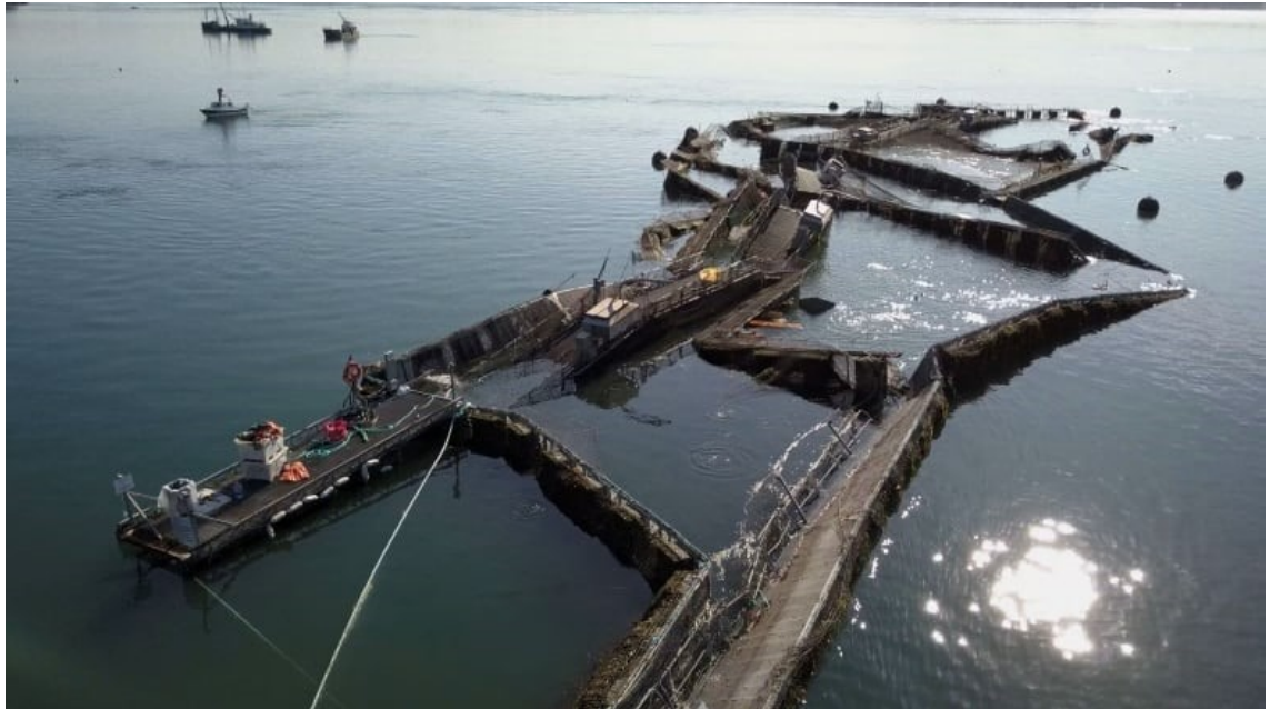
Figure 5: Collapsed aquaculture cages in Washington State facility (NB: these are steel rectangular cages; in Newfoundland the cages are circular and made of high-density polyethylene (HDPE). (picture by B. Garreau in McPhail, 2018)
