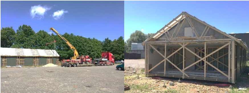
Figure 3-3. Separation and moving of the test building.
