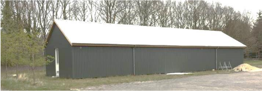
Figure 3-1. Picture of the full-scale test building at its first location.
