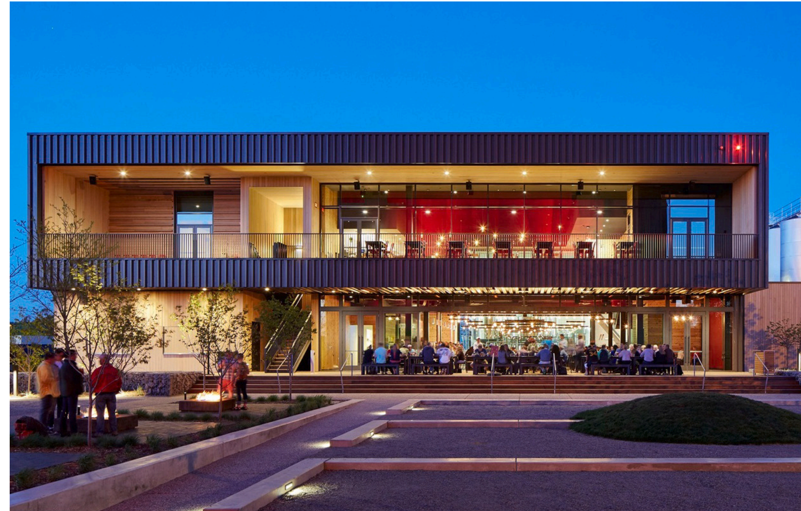
27.1 The concept of transparency runs through the entire project, and people can still see the activities of interior from outside.
