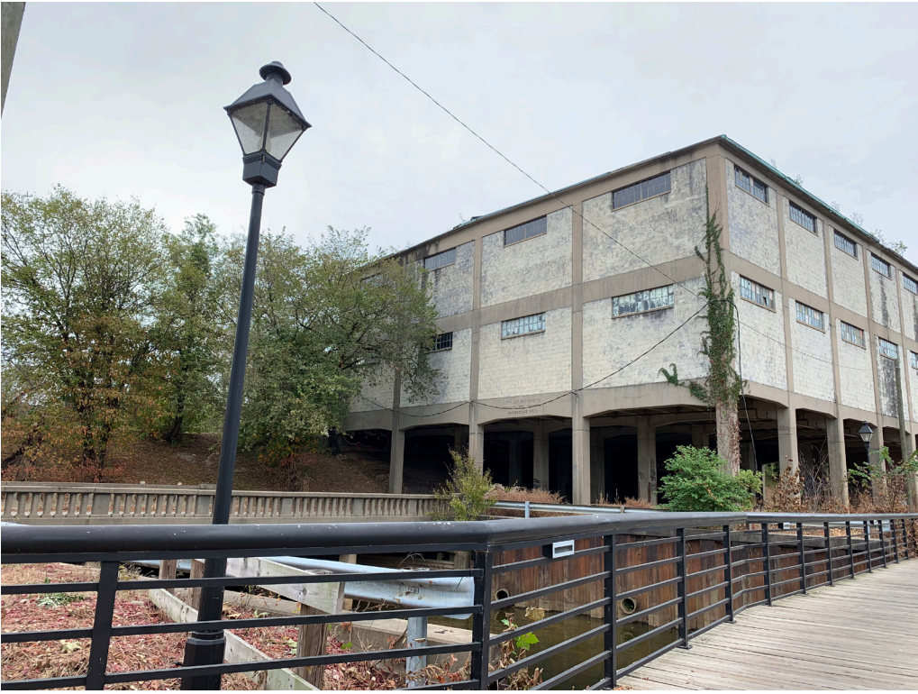
View B - From Bridge
