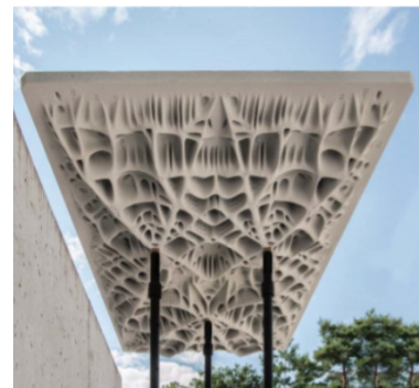
3D Printed Concrete Slab by ETH Zurich
