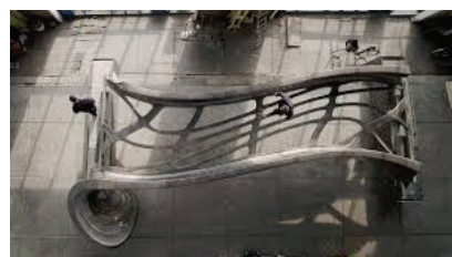
[figure 2.1.12] 3D Printed Bridge by MX3D
