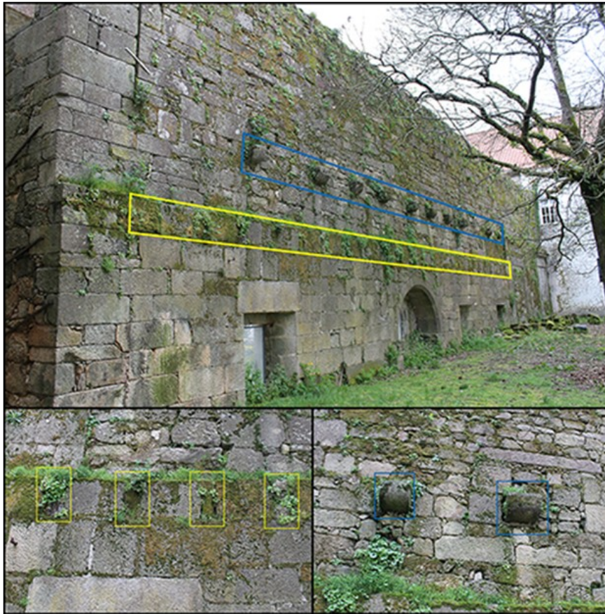
Fig. 9. Marks and evidences of the different systems from the first half of the 16th century (yellow) and prior to the second half of the 16th century (blue).
