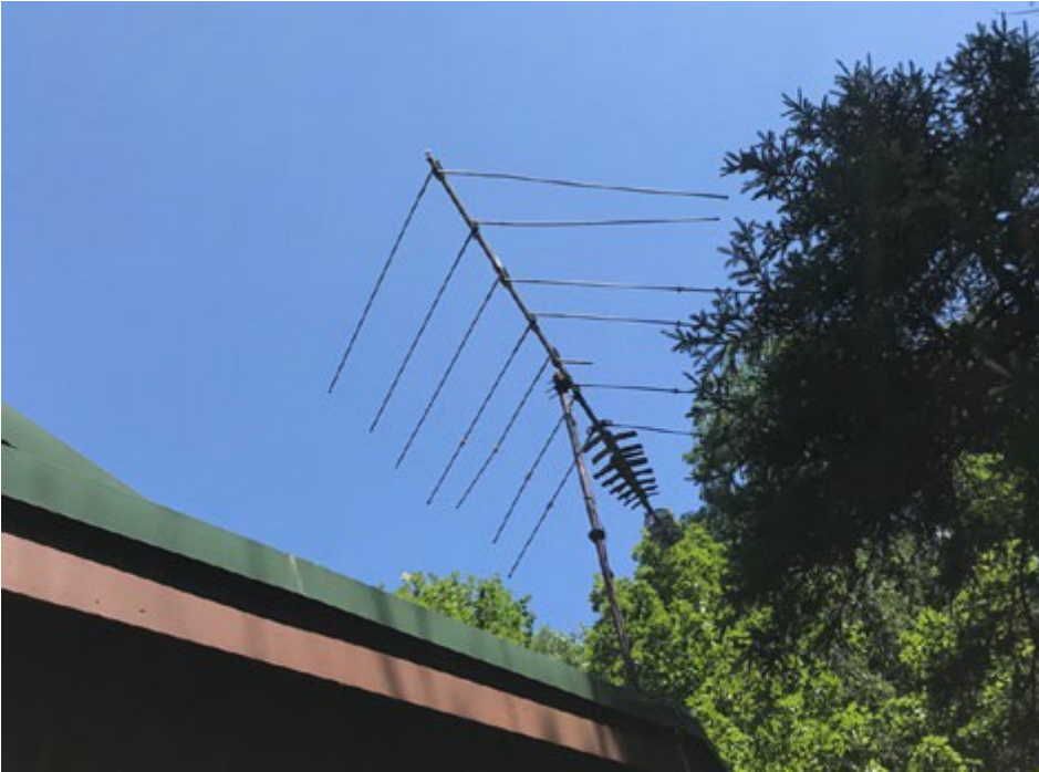
Figure 7. Television signal receiving directional antenna [2].
