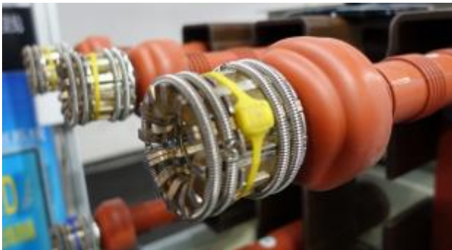
Figure 30 RFM3250 mounted using a flexible band [36]
