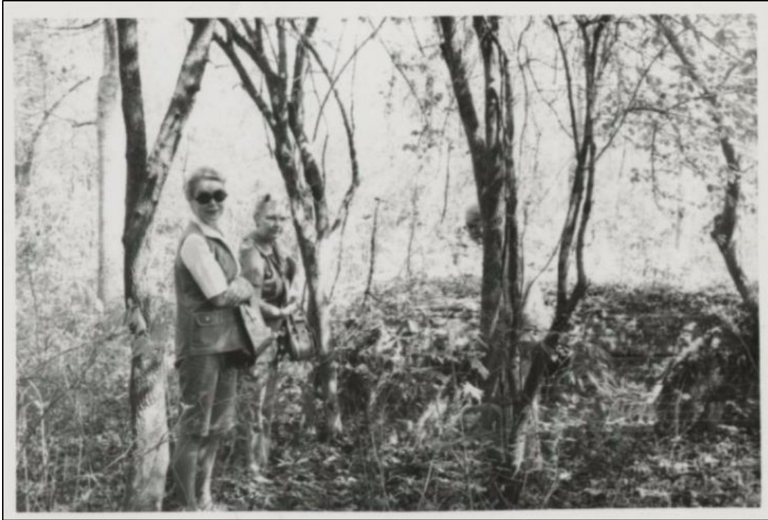
Figure 9: The ruinous state of the Gause Tomb in the 20th century from the “Horry County Historical Society Photograph Collection” at Coastal Carolina University.
