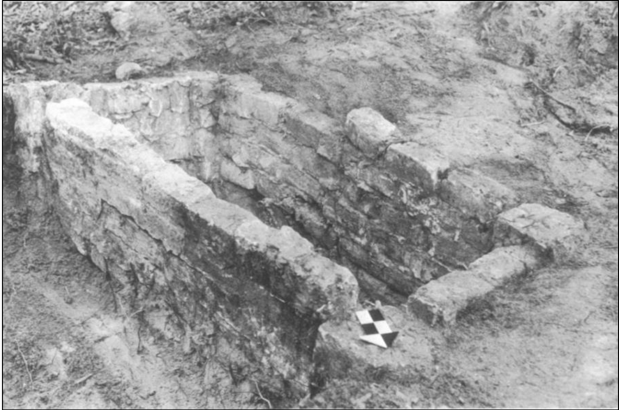
Figure 57: Found subterranean brick stanchion that was originally topped with flat ledger stone (from Thomas et al. 1977).
