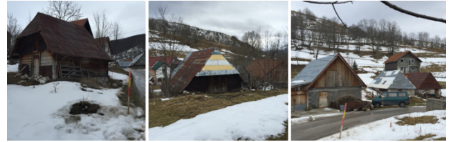
Figure 20: Some newly constructed buildings follow the patterns of traditional architecture
