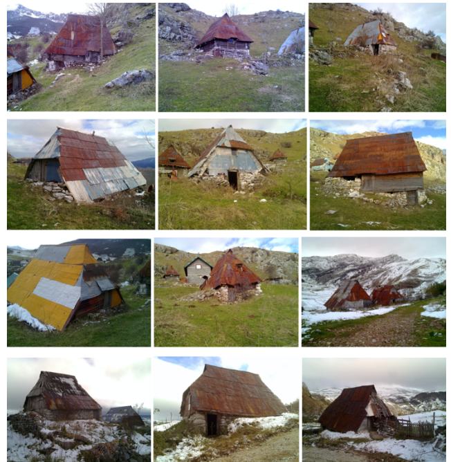
Figure 15: Katun settlement Gradina above Umoljan. Katuns preserved to this day
